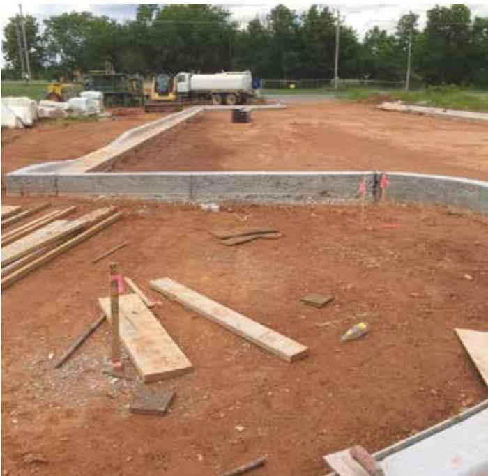
*Photo 1 – May 23, 2017, curb and guttering along east drive from McElroy entrance, looking north, by Mark Pruitt*
