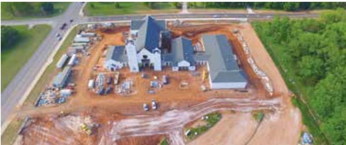
*Photo 1, aerial view of church site looking north, by Andy Arena and drone. Note on right side and bottom dirt work and soil stabilization (white lime) for drives and parking lots.*
