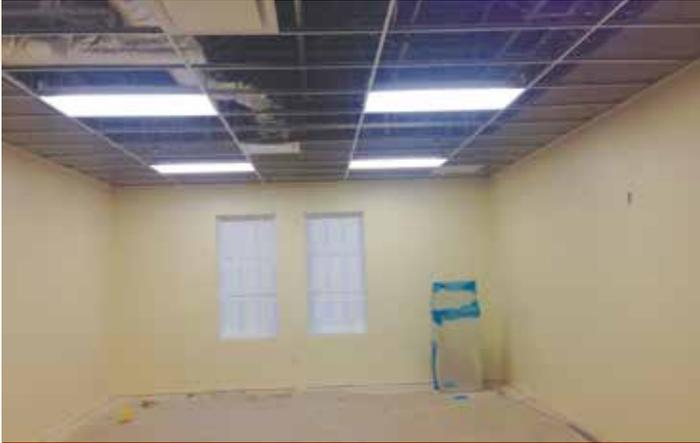
*Photo 7, finished wall paint, installed lighting, and HVAC supply diffusers, east classroom looking east, by Larry Hoberock.*
