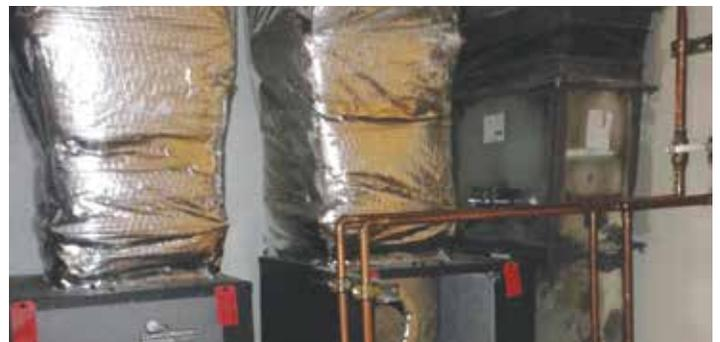
*Photo 6, HVAC units for ground source heat pump installed in mechanical room in education wing, by Larry Hoberock.*
