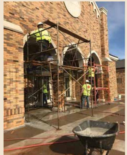
*Photo 10, Nov. 9, sidewalk and plaza at entrance to Parish Hall, showing washed gravel and regular concrete mix, looking northeast, by Mark Pruitt.*
