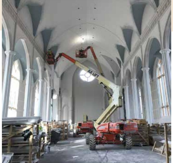
*Photo 4, Nov. 9, progress in nave, looking north, by Mark Pruitt. Note detail of GFRG frieze covering air conditioning supply vents, upper right and left.*
